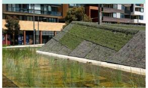
The Drying Green at Green Square, Sydney, has incorporated WSUD in the form of local wetland. WSUD can also be implemented through rain gardens, sediment ponds, swales and rainwater tanks.
