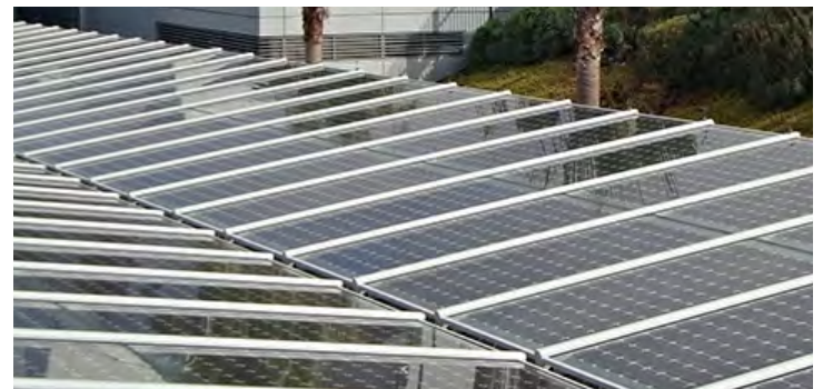
Photovoltaic solar shading structure to car park. 7
