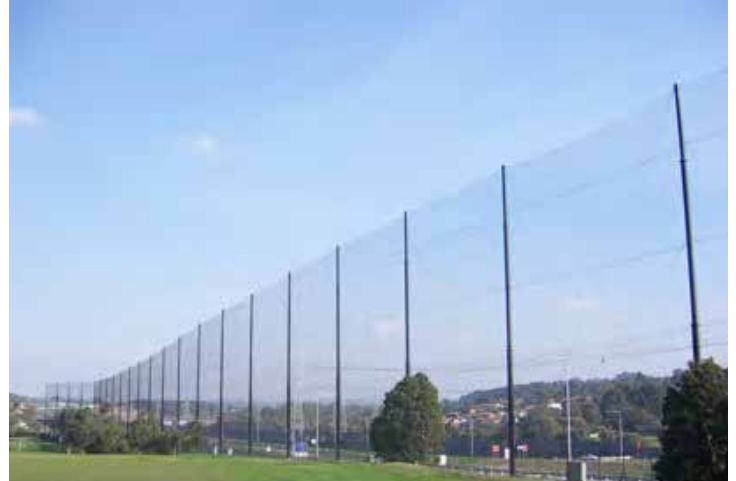
Low visual impact, high safety fence. Kevlar reinforced mesh, timber post supports
