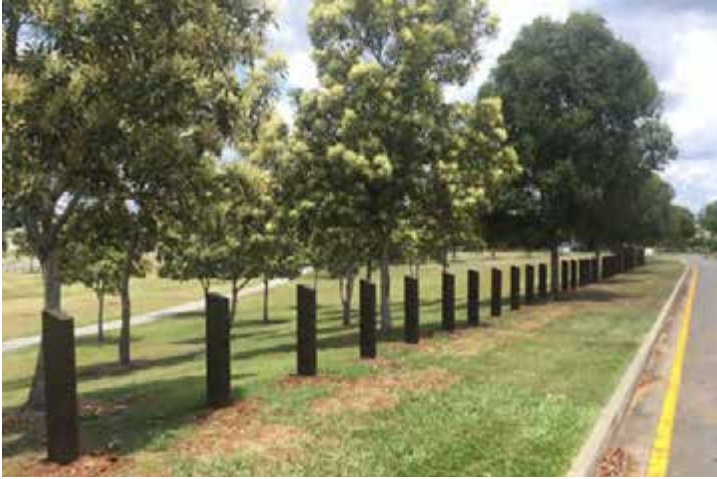
Timber bollard boundary fence type
