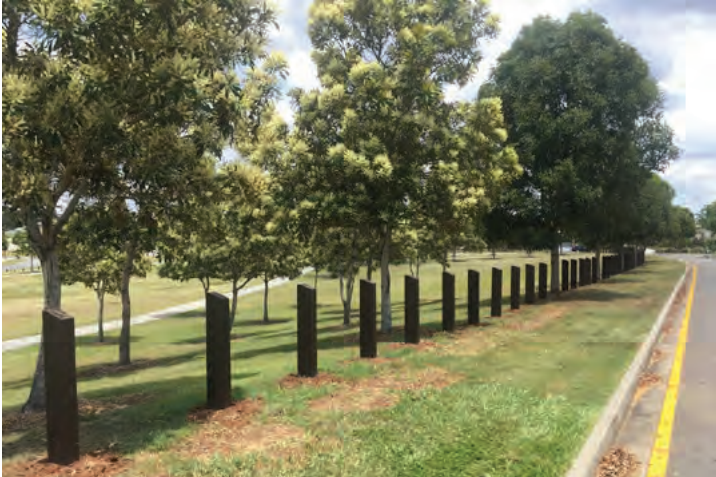
Timber bollard boundary fence type
