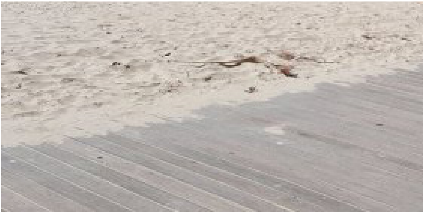
New timber deck with a flush finish to the sand 'beach'
