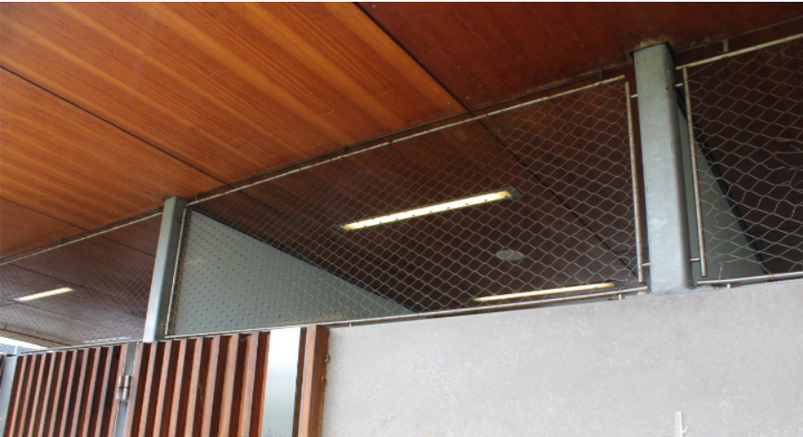
New toilets to have high external openings for natural ventilation and light
