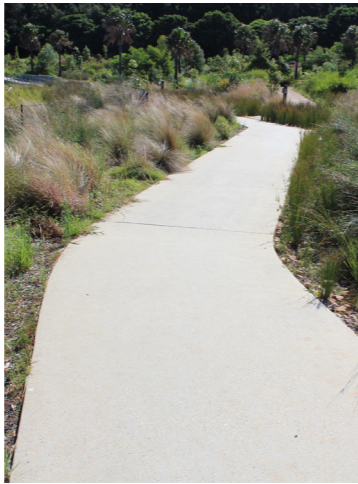
New 1.8m wide concrete pathway
