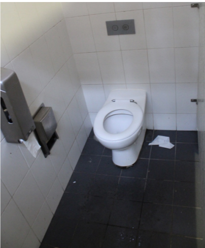
Concealed cisterns and stainless steel fixings to reduce vandalism
