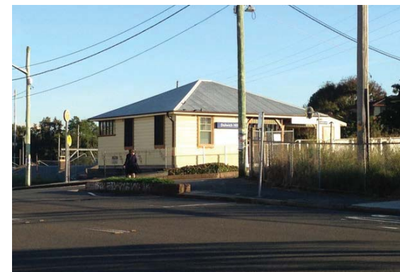
Dulwich Hill Station Ticket Office - timber weatherboard structure
