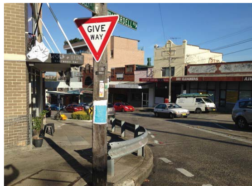
Adhock safety measures due to incompatibility between footpath width and required use
