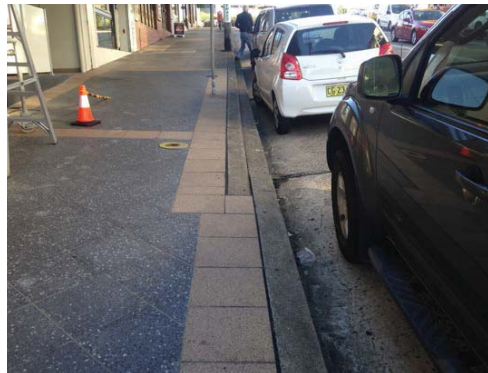
Steep grades and double height kerb- Wardell Road south of the train station
